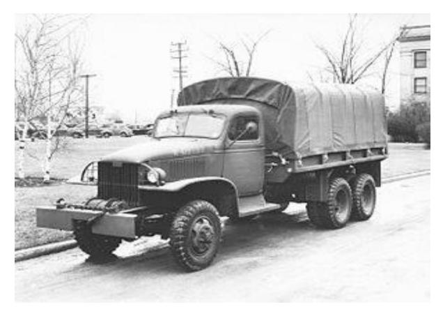
The truck most used in the Red Ball Express operation was the GMC CCKW, 2.5 Ton, 6X6
